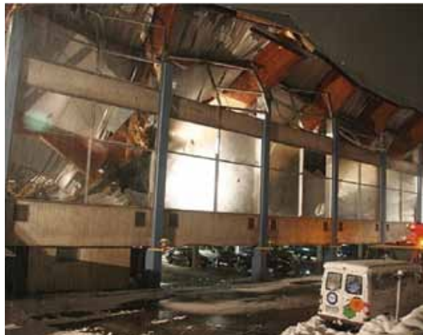
© M. Leitner, Collapse of the ice-skating arena in Bad Reichenhall
