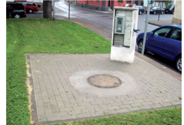
Remodelled well plant
