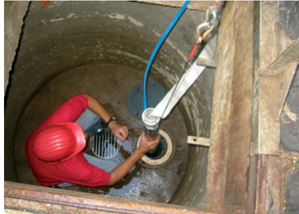
Installation of an submersible motor pump
