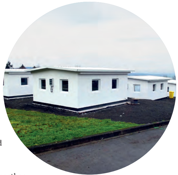
50 living space shelters for 6 to 8 people each were constructed in addition to sleeping accommodation in halls.
