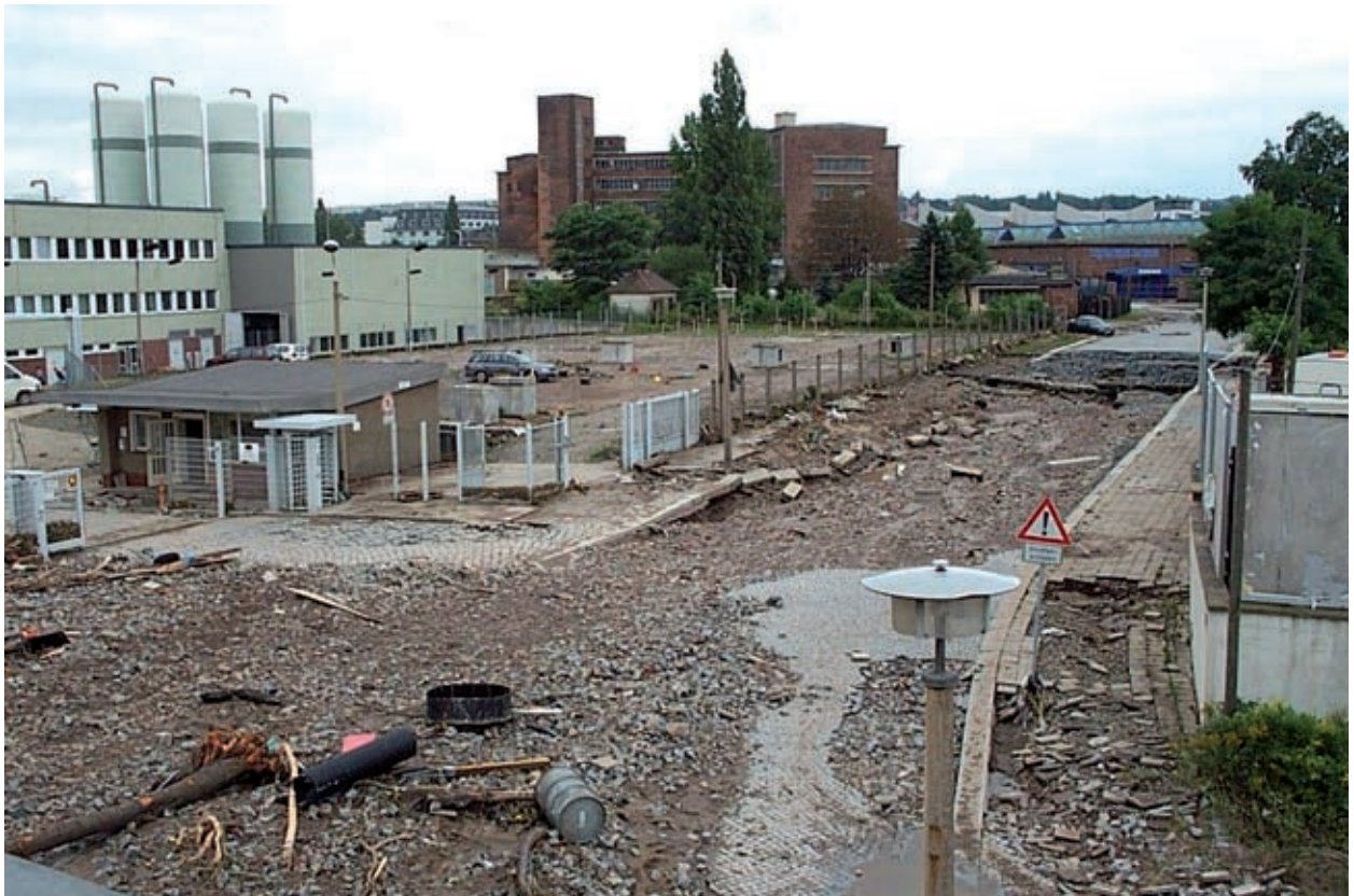
Figures 3.3 and 3.4: A flooding event occurring at Nossener Brücke power plant depot in Dresden whose legacy did not vanish without trace after the waters receded
